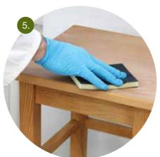
After the first coat of the lacquer we sand the surface with a sanding brush or sanding paper of granulation 280 - 320. Then follows the second coat of lacquer and drying at room temperature (18-22°C and relative humidity 55-65 %).
